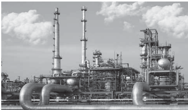
PX unit at Panipat Refinery
