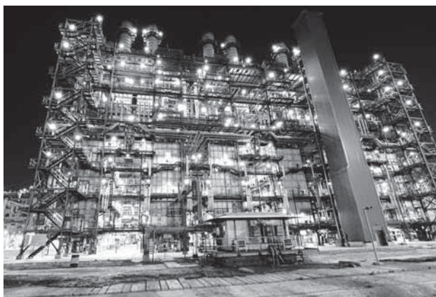
A view of Naphtha Cracker Unit at Panipat
