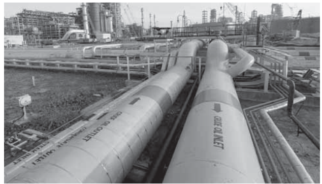
Crude Oil Pipeline at Paradip Refinery
